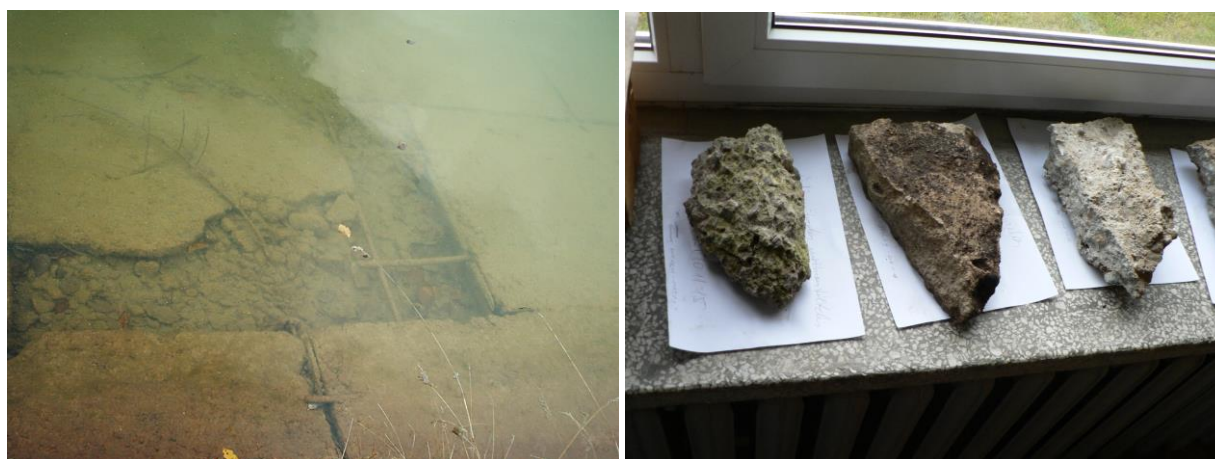
Fig. 3 Samples from reinforced concrete strengthening slabs in Graužė hydroscheme
