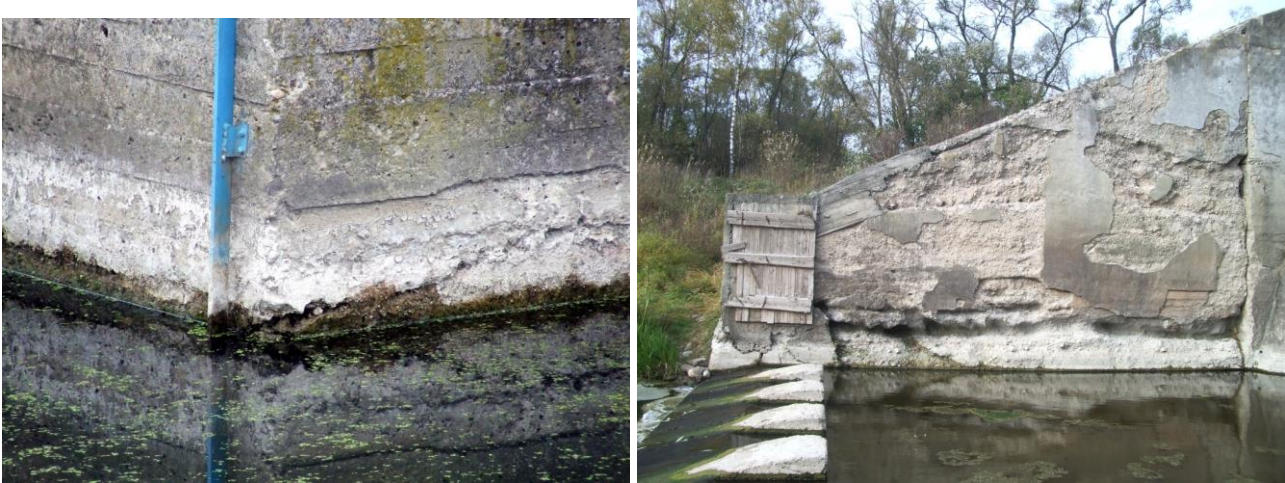
Fig. 1. Propagation of corrosion of concrete
