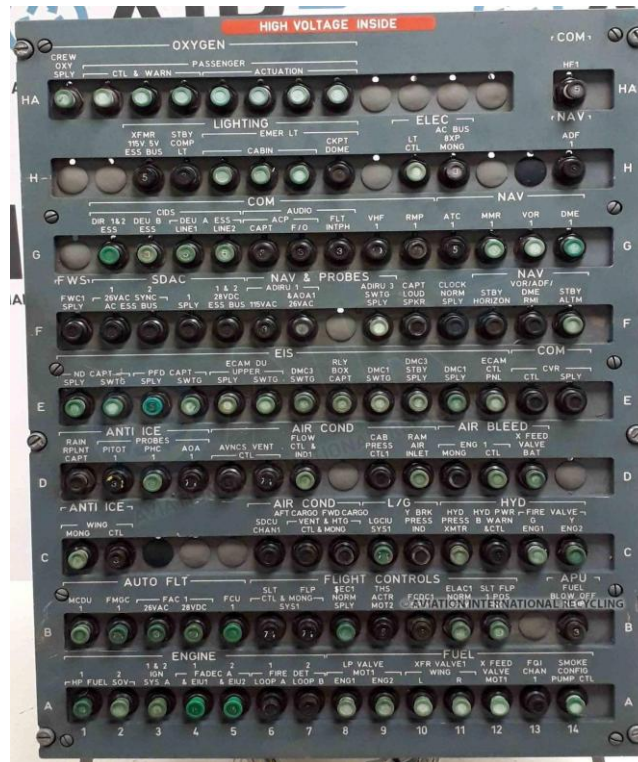
Fig. 4. A330 Secondary Circuit Breaker panel [4]
