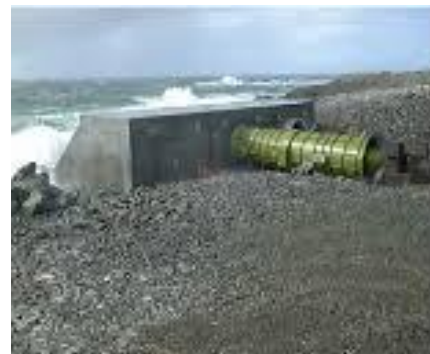
Fig. 3. Prototype of Oscillating water columns (OWCs) [1]
